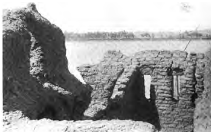
(b) View at roof level from northeast.
